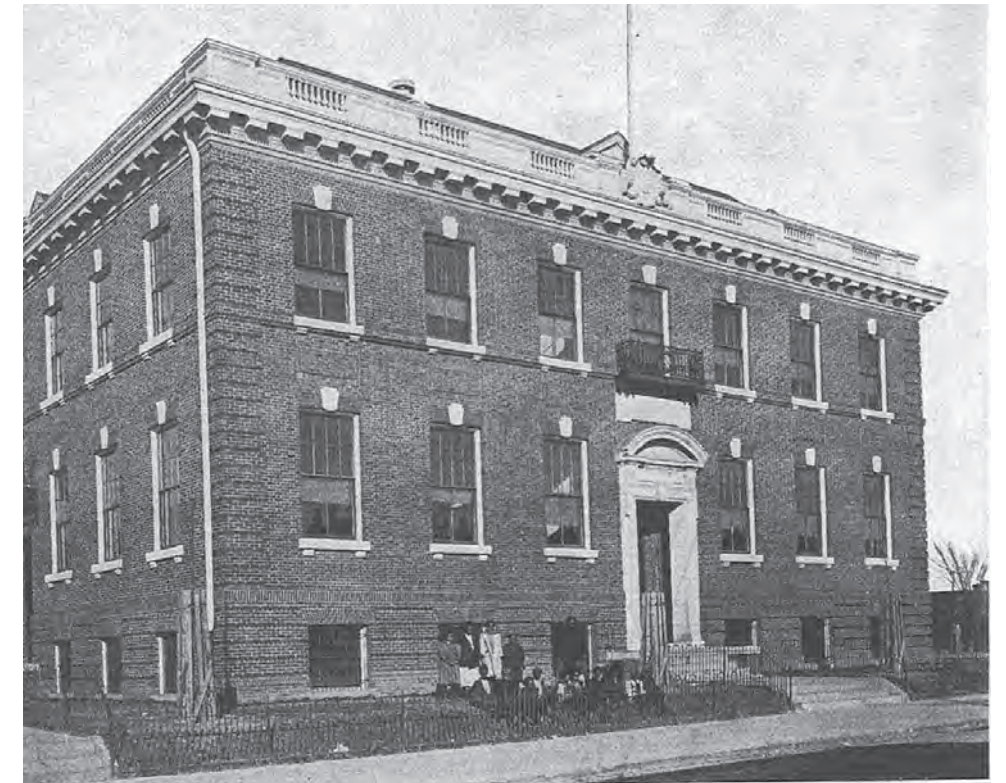
CENTRAL BUILDING PHOTOGRAPH (1908)- ROLLED CURB
