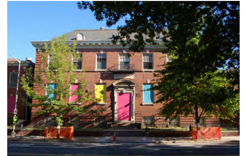
SOUTH ELEVATION (EXISTING CONDITIONS)
